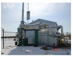
Figure 15 - Natural Gas Fired Heater
